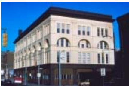
Building is located at 702 Monroe Street corner of Ontario.
